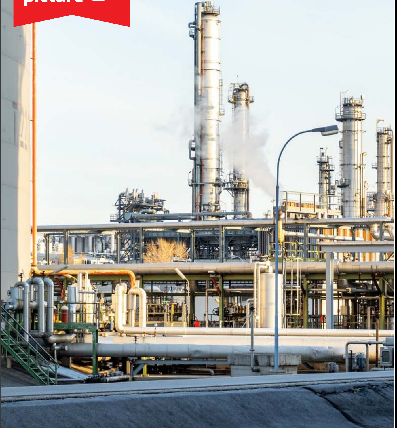
■ Port Harcourt Refinery Rehabilitation
